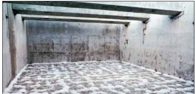
Better air scour action – and better media cleaning – is the result of closely spaced, non-clogging orifices and uniform distribution of air throughout the length of the underdrain lateral.
